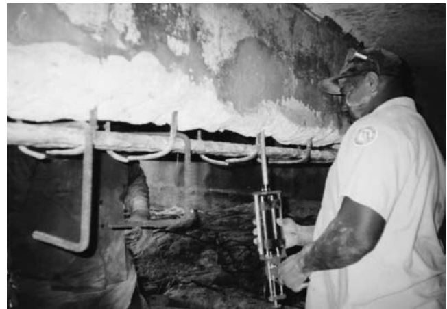
Figure 3.7. Epoxy injection of cracks.
