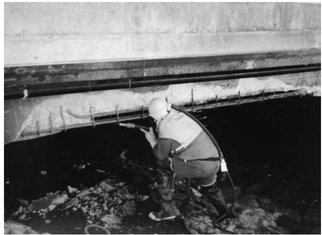
Figure 3.2. Sandblasting of corroded steel.
