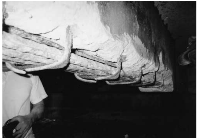
Figure 3.3. Splicing of damaged bars.
