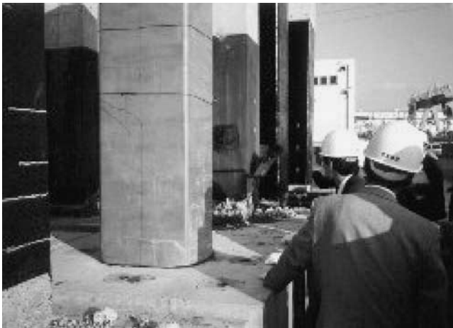
Figure 3.8. Column wrapping.
