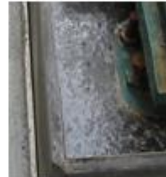
After removing the formwork, all flanges are chamfered
