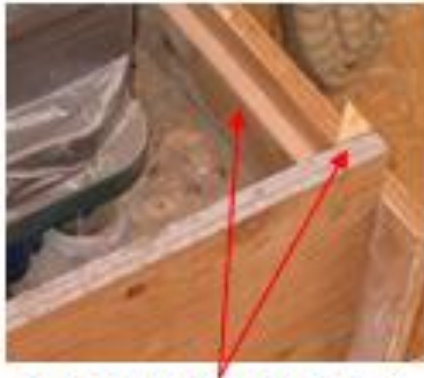
Wooden triangle slats which are installed in the formwork
