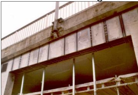
Shear & Flexural Strengthening
