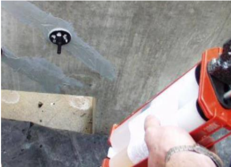
Structural Crack Repair by Epoxy Injection (ACI RAP-1)
