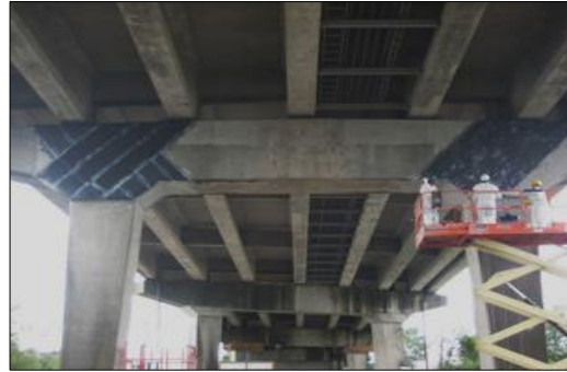
Shear Zone Strengthening
