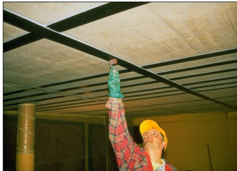
Flexural Strengthening & Deflection controlling
